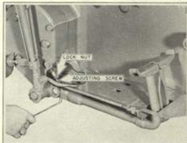
Figure 7-8 Adjusting Disc Brakes
