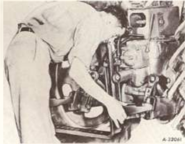
Illustr. 27 Installing the drawbar.
