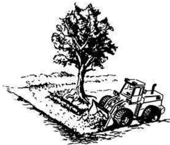
Fig. 4.41. Removing Large Trees
