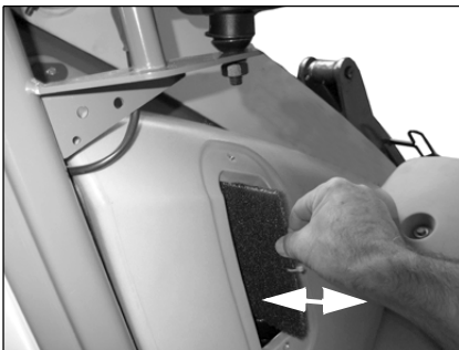
Fig. 183: Replacing the dust filter of the heating system
