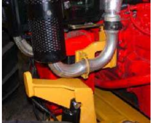
Replacement Exhaust Pipe Installed
