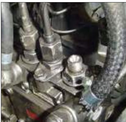
Fig. 8: Opening on fuel pump
