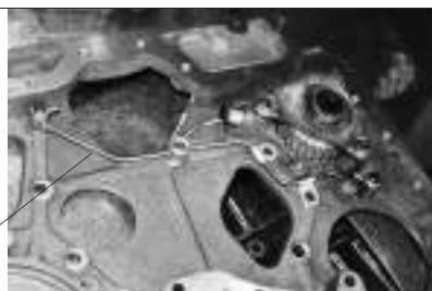
Fig 5-24 Lubricating Pipes Installation
