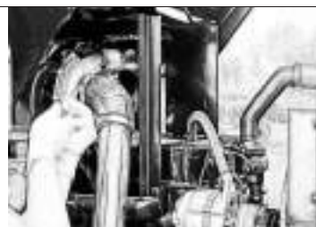
Fig 5-32 Connecting of Intake and Exhaust Pipes
