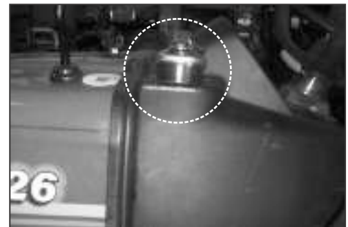
Diesel Tank Cap for Filling Diesel
