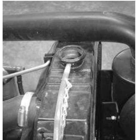
Picture 4-33 Engine Cooling System Maintenance
